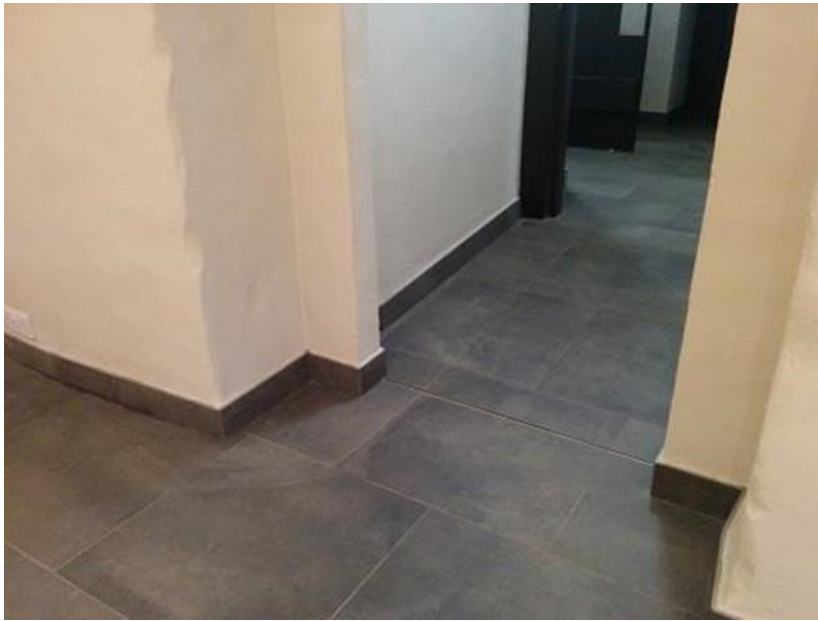
Image 15: Upwards slope to toilets
