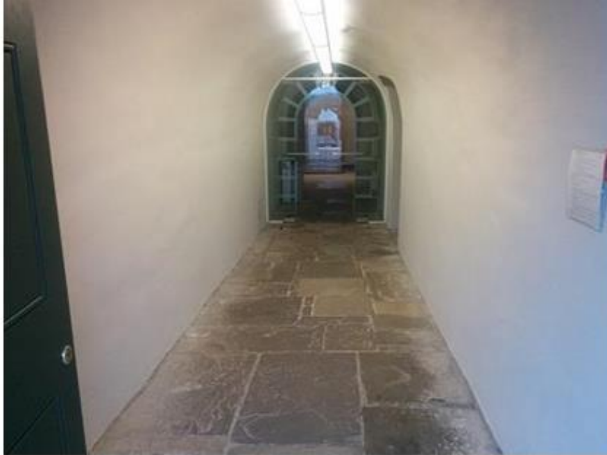
Image 16: Downwards slope into Undercroft
